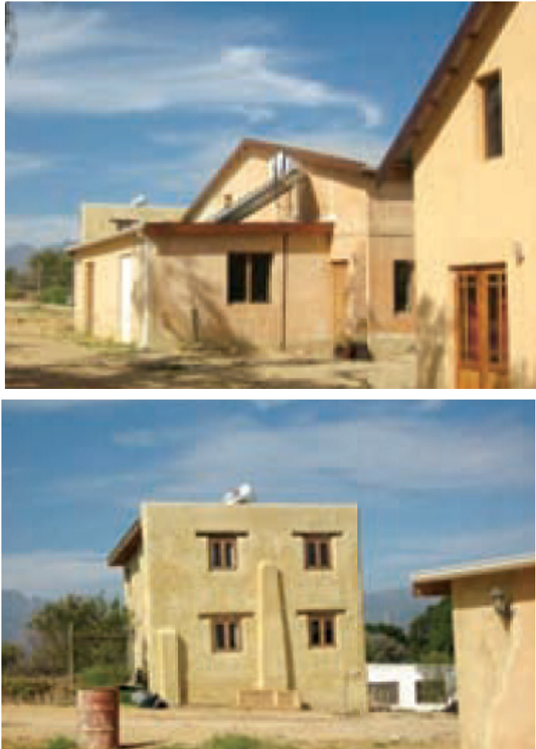
Figure 2.4: Adobe brick homes in Lynedoch, Ecovillage (a), luxury double-story house in Lynedoch, Ecovillage (b). Photos by Pierre Roux [62]
