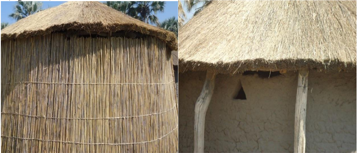
Figure 14a and 14b reed and mud hut showing eaves in Shakawe (Photo: Courtesy of Barbara Ngwenya)
