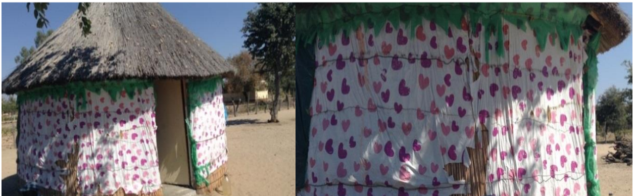
Figure 14c: house screened with plastic material, structural adaptive strategy in Shakawe (Photo: Courtesy of Dirontsho Maphane)
