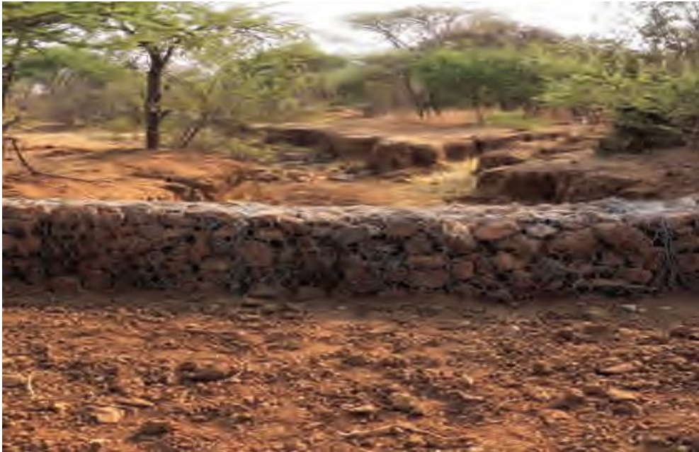
Figure 2.1: Gabions for soil erosion control at MNR: Source (MWF Booklet, 2014/15)
