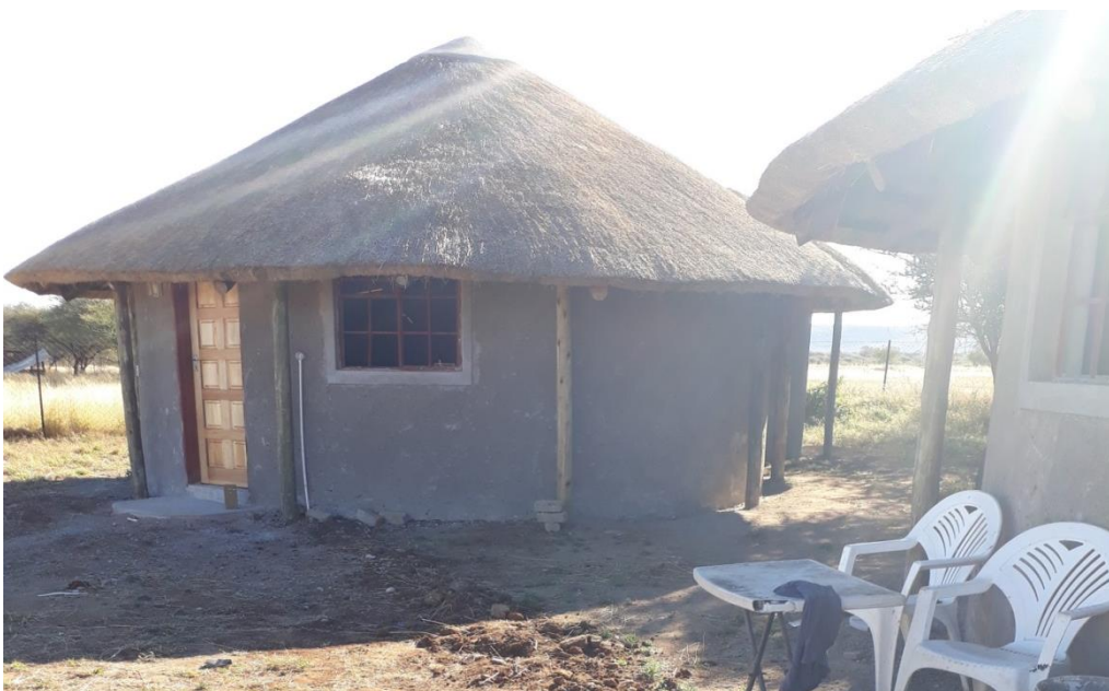
Figure 4.10 Mokolodi Village Guest House under construction (2018). Photo: J. Maradza
