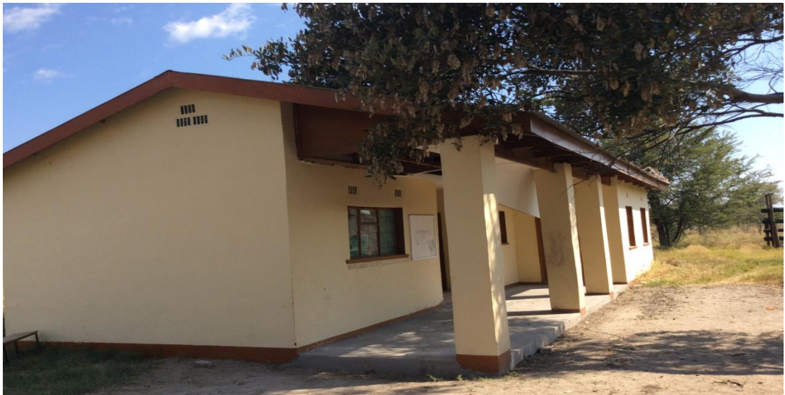
Plate 2: Sankuyo Tshwaragano Management Trust offices (one of the CBNRM projects at Sankuyo village)
